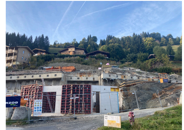
Picture 1: Site location
