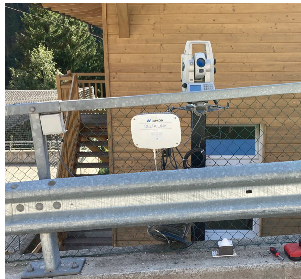
Picture 3: Total station and Senceive Triaxial Tilt Sensor Node
